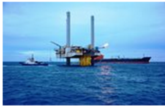
Oil gas and marine industries to benefit from the services provided by Trinity's new division
